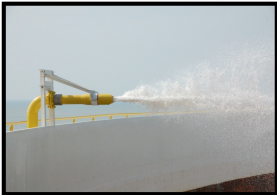
Gambar 4.13: Full surface foam system
