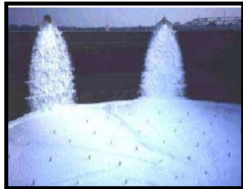
Gambar 4.14: Full surface foam system
