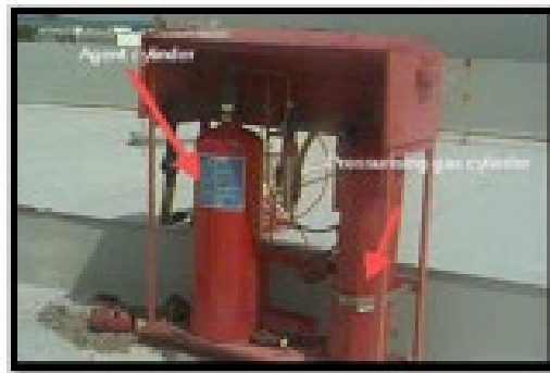
Gambar 4.14: Full surface foam system
